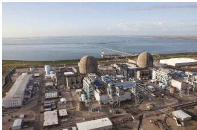
South Texas Nuclear Project near Houston
